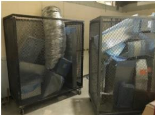
Large bins can be used for duct fittings
