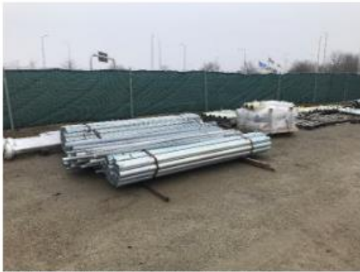
Exterior materials stored on dunnage
