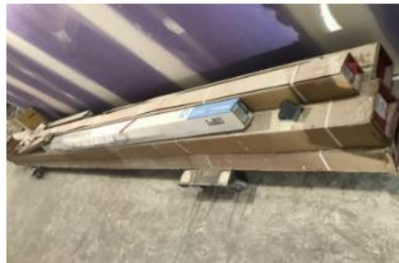
Long materials (i.e. ceiling grid/handrails) stored on dollies
