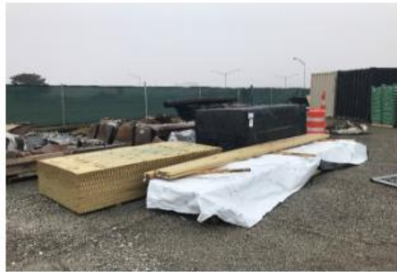
Exterior materials organized and properly stored
