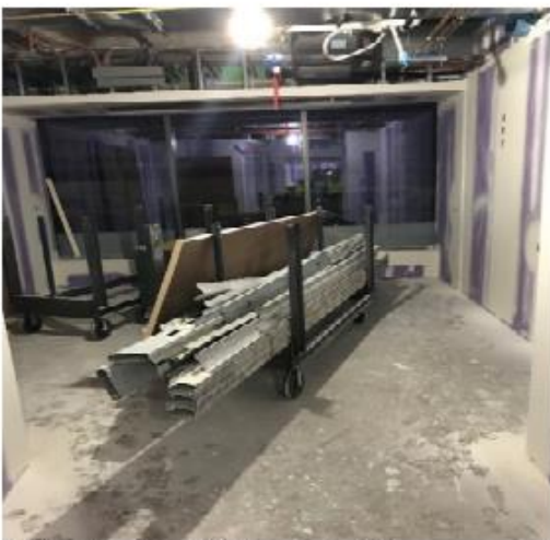
Pipe racks for miscellaneous studs
