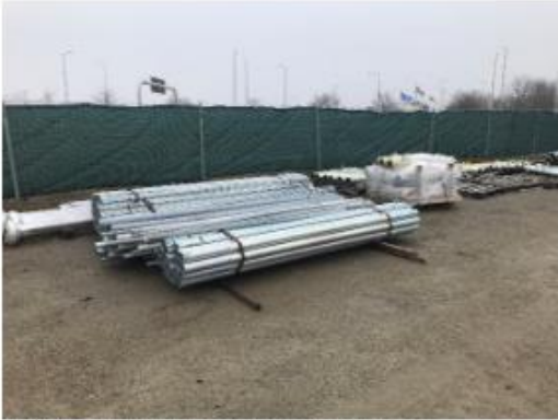
Exterior materials stored on dunnage
